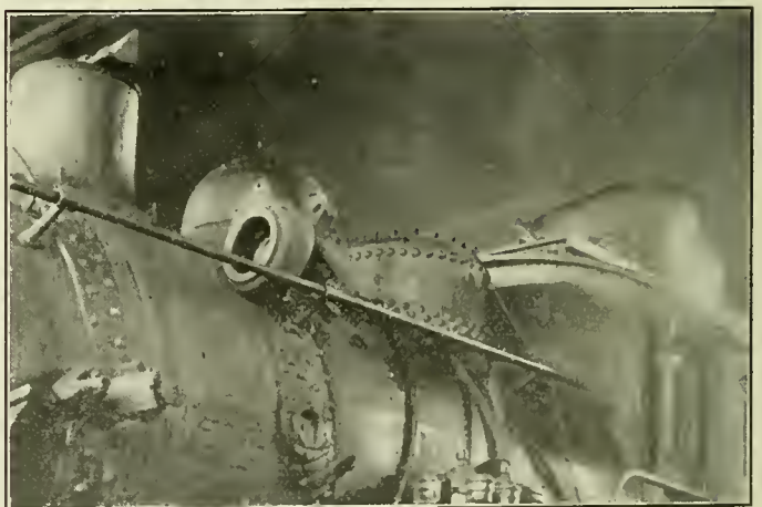
Dismantling of Dome Required to Regrind Dry Pipe Connection
